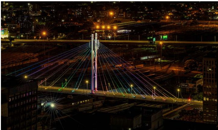
Mandela Bridge by Belinda Ueckermann
