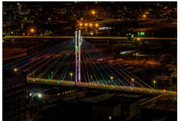
Mandela Bridge by Belinda Ueckermann
